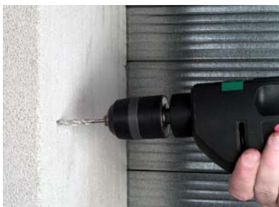
1. Perforar la pared
