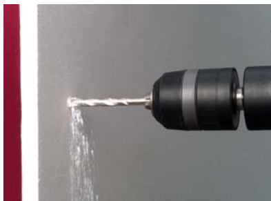
1. Perforar la pared
